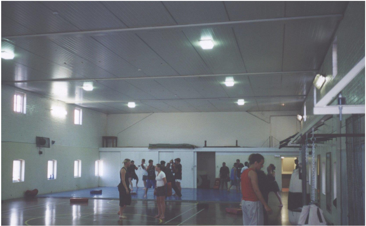
The new insulated ceiling in the McKenzie Gymnasium helped with heating, lighting and acoustics. Crichton Cobbers' Club.
